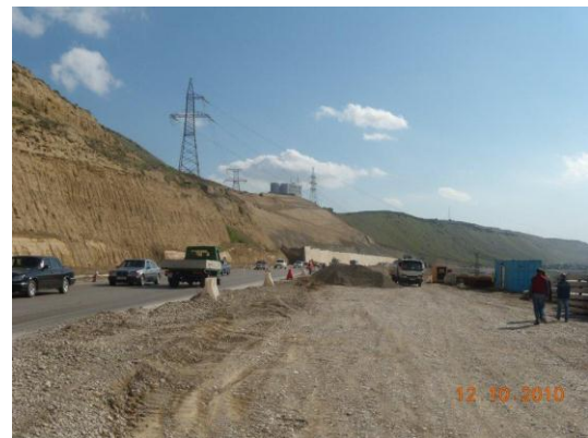
Fig. 6b. Cut slopes-Existing Highway Lanes
