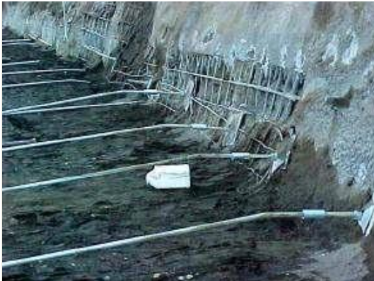
Fig. 4. Direct Connection with Steel Rods
