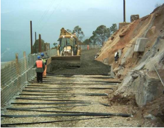
Fig. 3. Direct Connections with Synthetic strips
