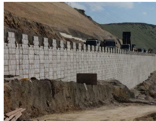
Fig. 10. Construction Phases – Panels and RE Wall
