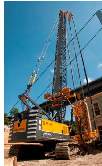
Figure 8. Diaphragm Wall Machine, Hydrofraise-Cutter
