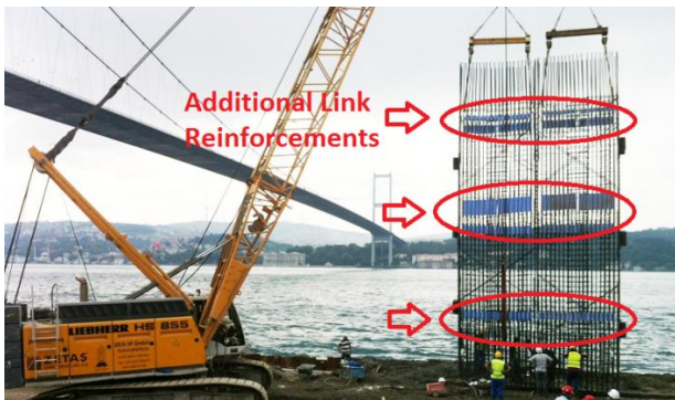
Figure 11. Additional Link Reinforcements on the Slab Elevations
