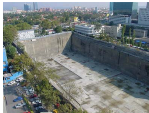
Figure 3. A photograph from Kanyon Complex
